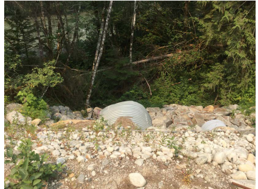
Looking downstream from road surface
